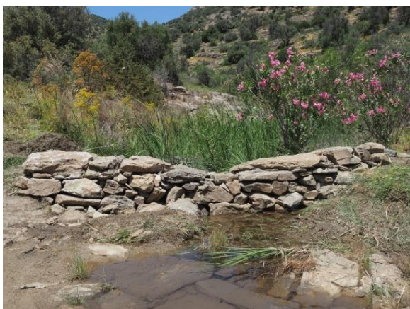
A traditional stone check dam on Kavouropotamos stream on the island of Paros, Greece. Photo: Thanos Giannakakis, WWF Greece
